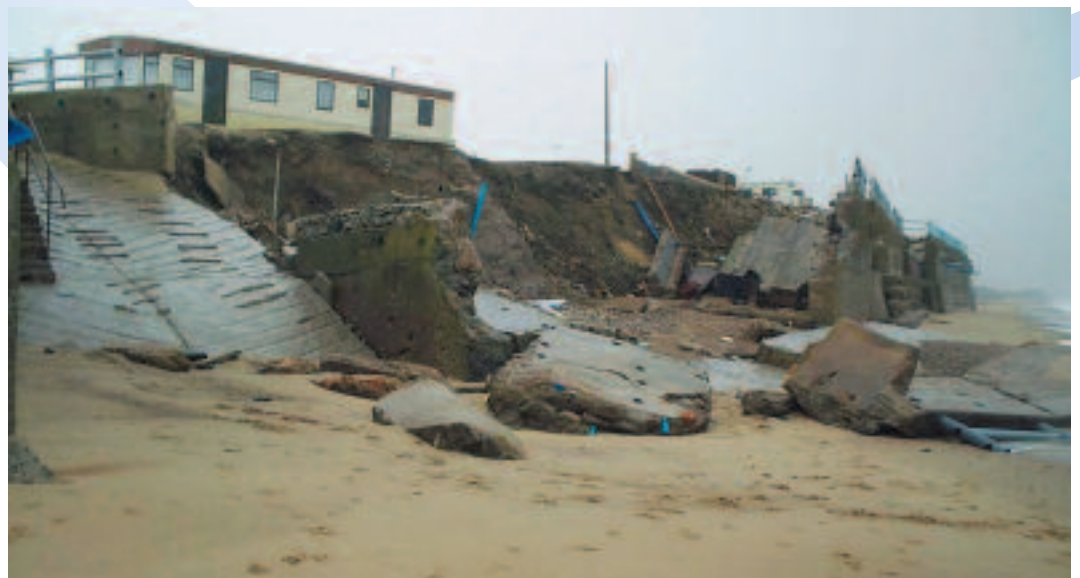
Failure of private defences at Ulrome, spring 2004
